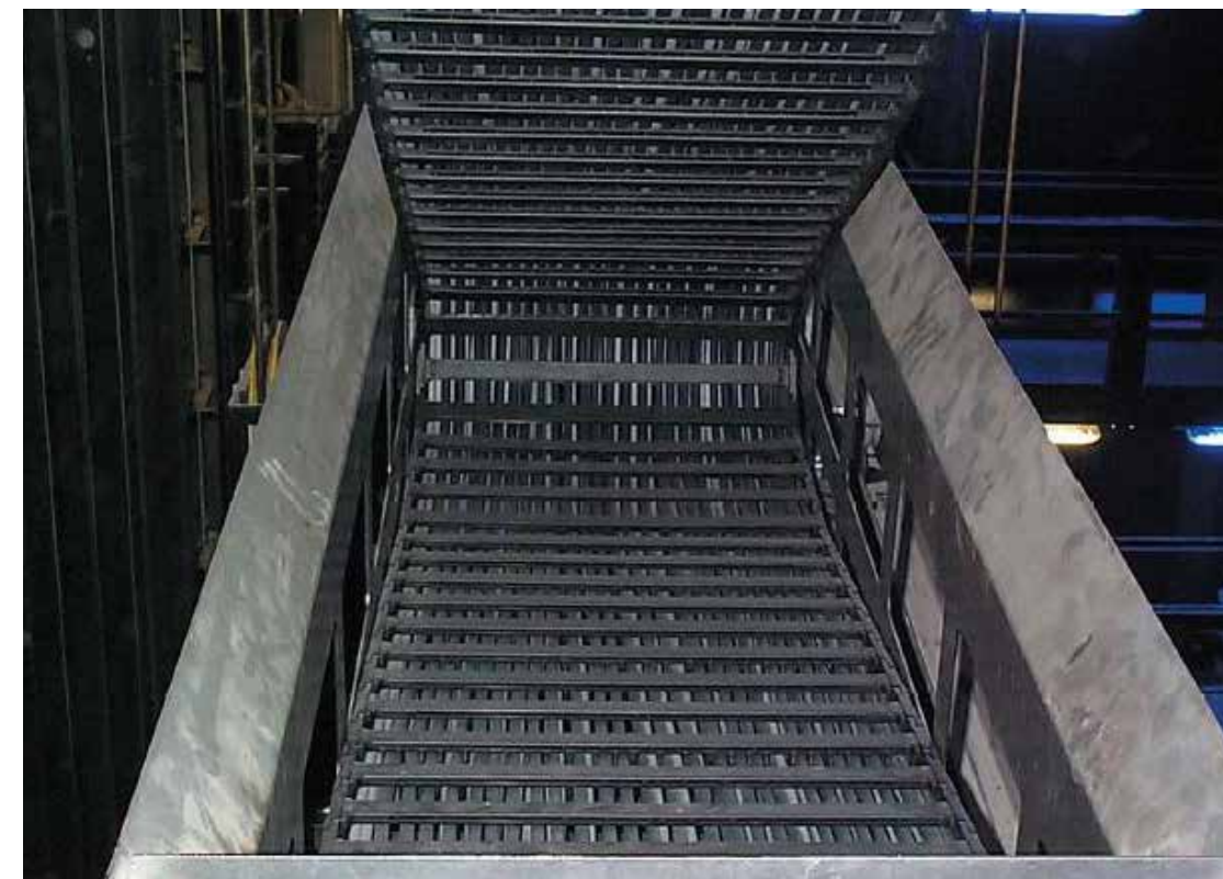
Coax cable and other chainflex® cables in a stage technology application. e-chain®: E4/4 system
