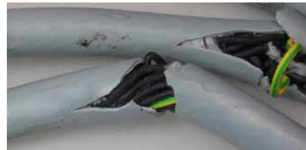
Jacket damage after 41,000 strokes ...
